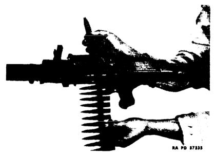
Figure 21 - Loading Machine Gun with Belt
