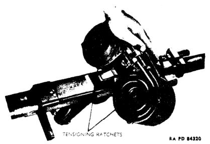
Figure 27 - Mounting of 75-round Magazine
