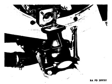
Figure 154 – Installing Governor Assembly
